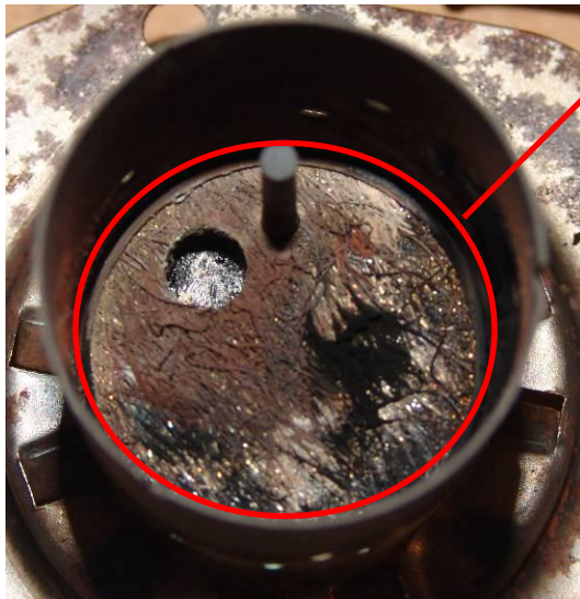
Inspect burner mat
